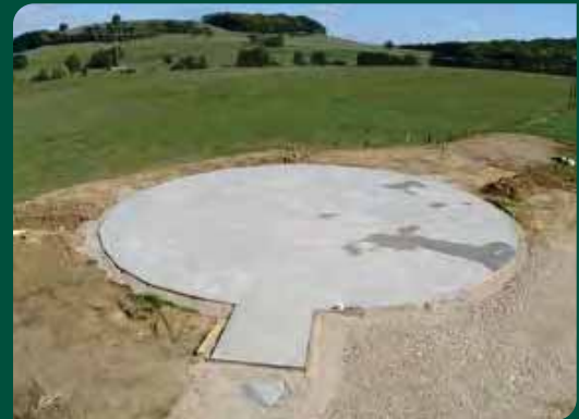
On-site base plate
